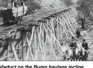
Viaduct on the Bump haulage incline one of the many tram lines built and used by the Australian Seasoned Timber Company.
